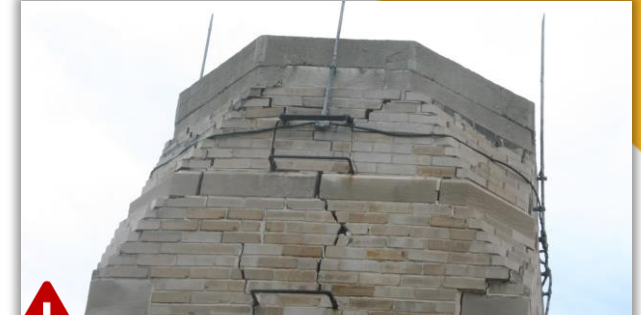
Displaced Chimney Masonry
