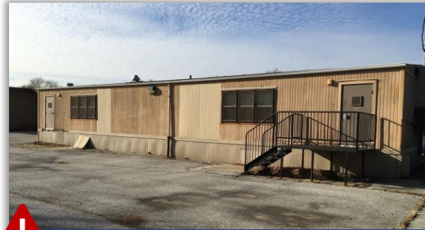
Existing modular building
