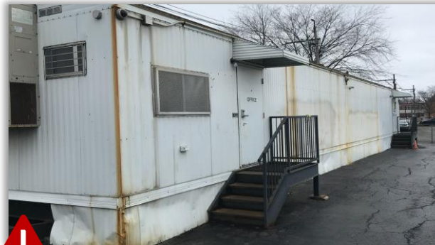
Existing modular building
