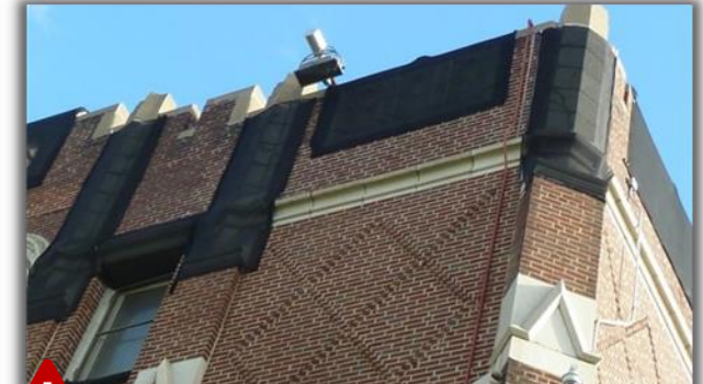
Temporary stabilization of brick erosion
