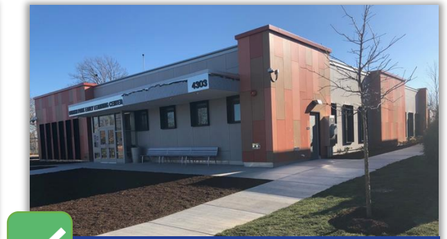
New/Replacement modular building
