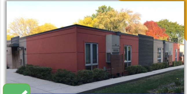
Replacement modular building
